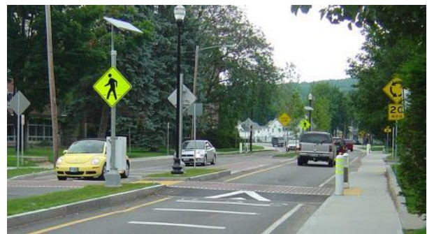
An example of a raised crosswalk.
