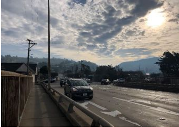
The Manor Drive overcrossing.
