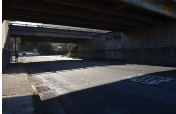
The Clarendon Road underpass.
